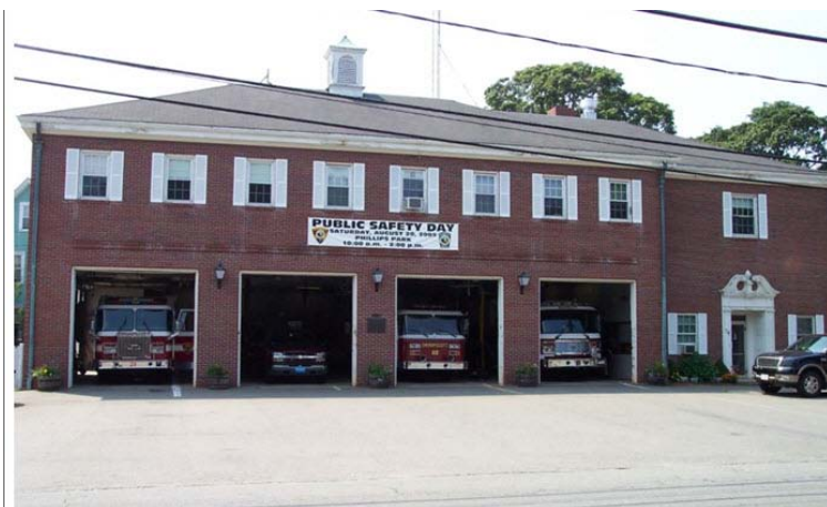
Swampscott Fire Department 76 Burrill Street
