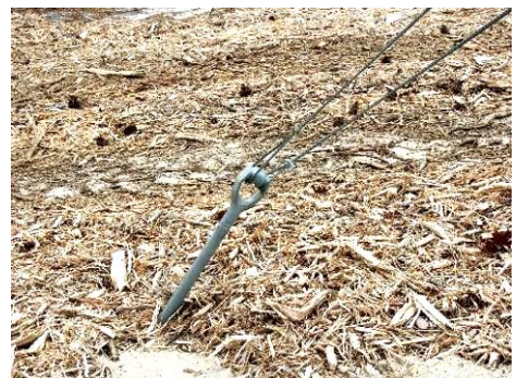
An anchor, installed, with 2 guy wires attached
