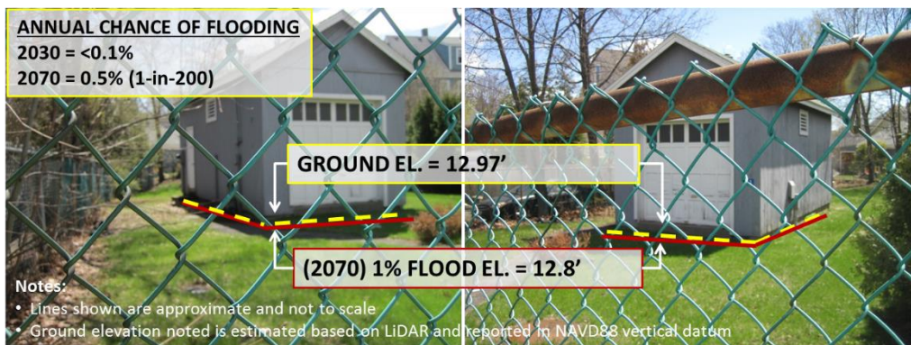
FIGURE 3.28 CHLORINATION STATION FLOOD RISKS
