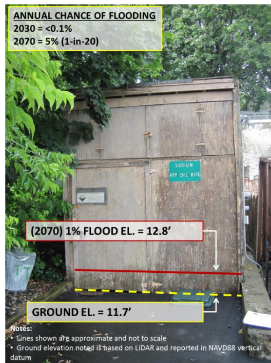
FIGURE 3.28 CHLORINATION STATION FLOOD RISKS
